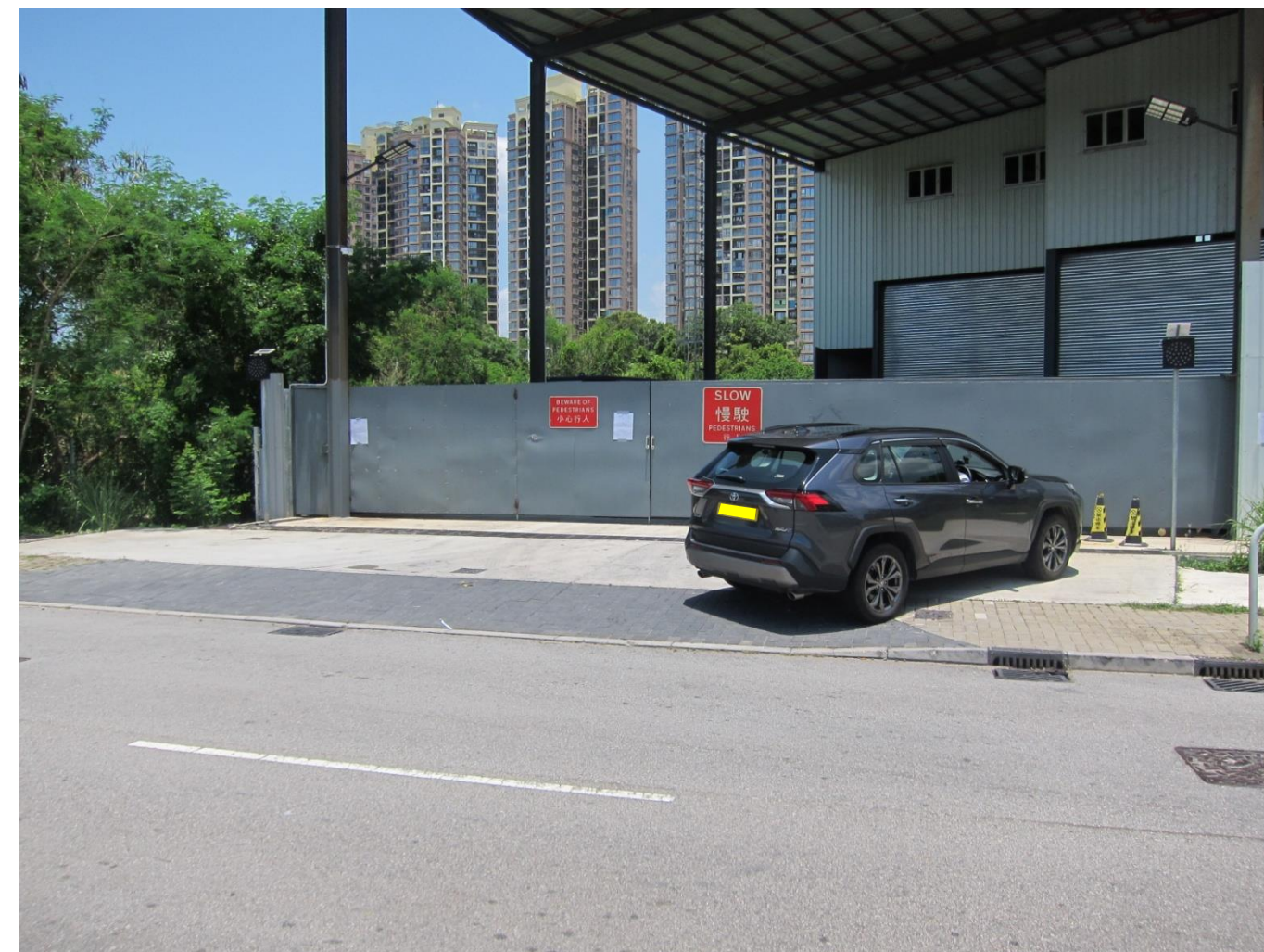
Revolving lights at the entrance
