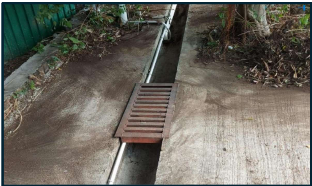
Typical Steel Grating on existing U-channels
